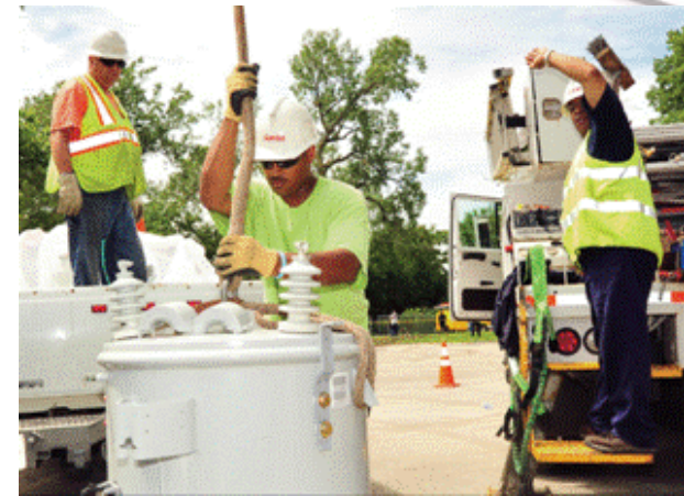
Workers on Chicago's south side replace a damaged transformer.
