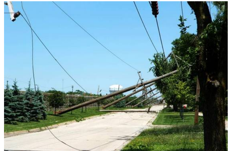
28 fallen transmission poles in DesPlaines
