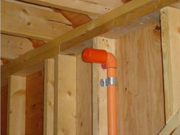
possible try to keep the sprinkler pipe in "warm space". Unfortunately, with residential sprinklers, it is sometimes necessary to run pipe in the attic. When sprinkler pipe is run in an attic, certain precautions must be taken.
